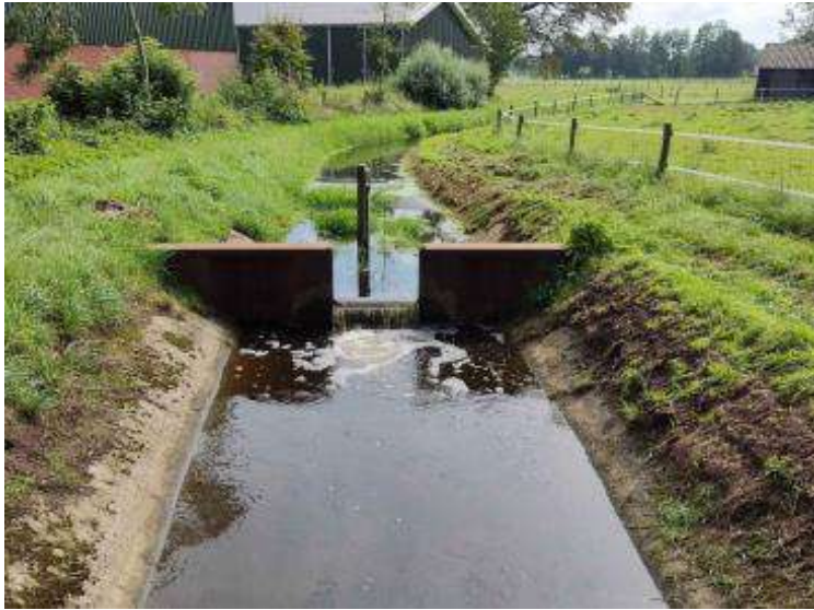
Figure 2: Example of a weir.
